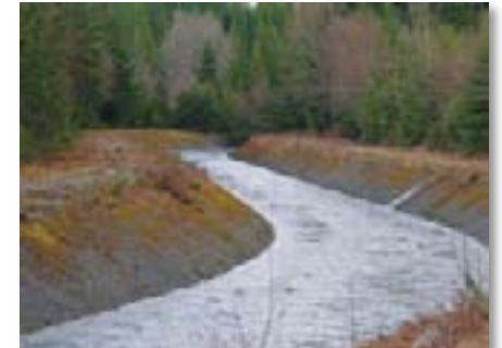
A portion of the water from the Salmon River is diverted through this concrete sluice into the upper Campbell River system to enhance the hydroelectric capacity of the John Hart Dam.
